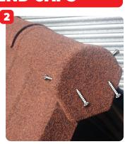
Screw through the end cap AND ridge tile into the batten. Optionally, screw through the face of the end cap, through the dry verge and into the batten.
