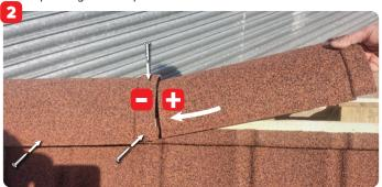
2 Set the first ridge tile into place, ensuring a neat overlap of the tile below. Interlock the *male* end (+) of the ridge tile into the *female* end (-) of the first ridge tile, and screw into the woodwork.
