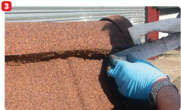
**TIP:** If the Flexim sticks to an area that it is not required, use a ball of Flexim to unstick the unwanted Flexim (like a ball of Blu Tack).
