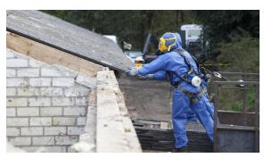
this reason the respirator is always the last item to remove when the job is finished. This person will have to remove the respirator before removing his blue coveralls which no doubt will contain asbestos fibres.
