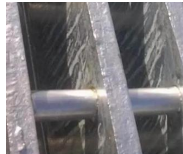
Swage-Locked Grating
