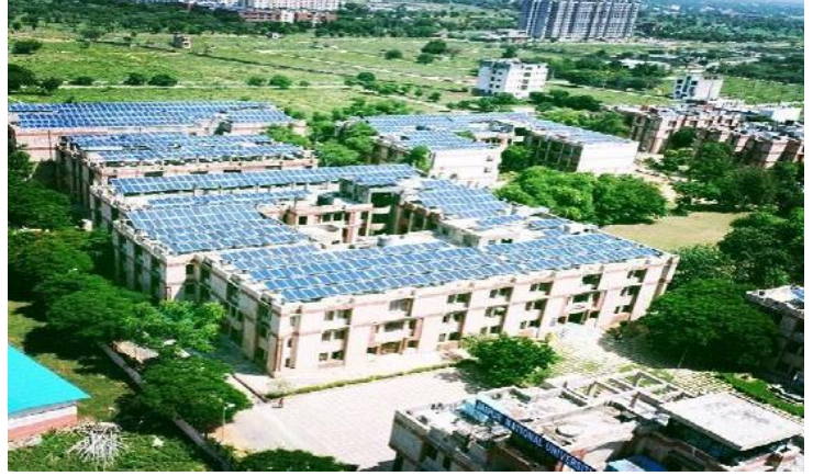
600 kwp Rooftop Jaipur National University, Jaipur
