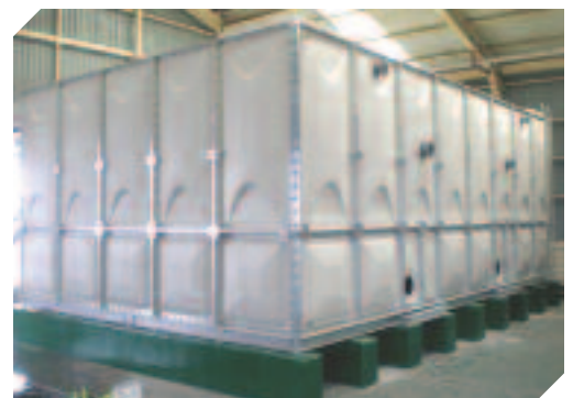
Completion of Installation Assemble panels with steel reinforcement members on site
