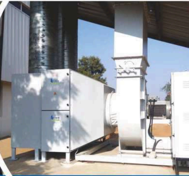
Outdoor installation of fume extraction system
