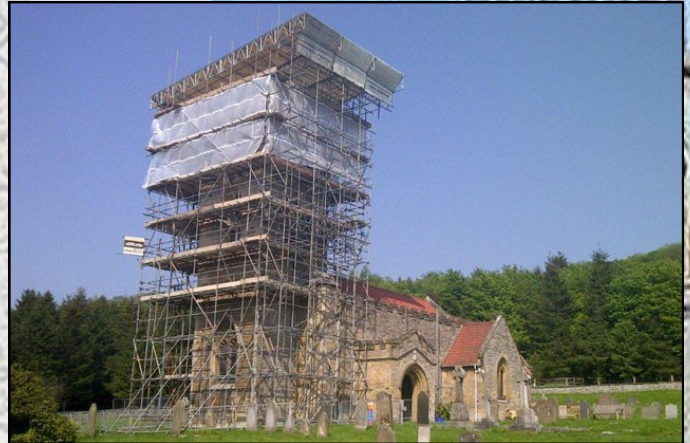
Picture by: Altitude Scaffolding.
