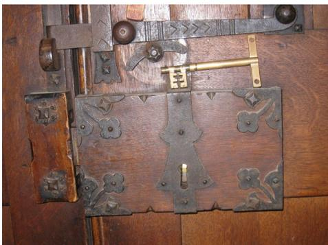
**Modern bronze replacement key for use on an 1890's stock lock. Not pretty, but functional. This lock is still in service, but this is not a final exit door – there are also bolts on the inside.**
