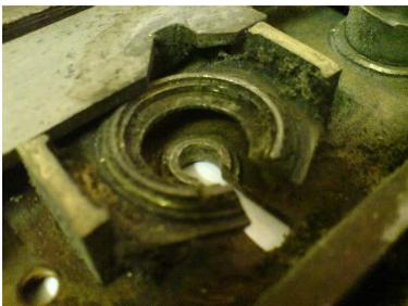
**Bridge ward clogged — needs cleaning; GT85 and toothbrush will shift most of this. The talon (notch) of the bolt tail is visible above the bridge; the tumbler is unseen below it.**
