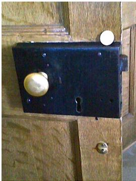
**19C 3-bolt rimlock (the coin is a £1). The practice of painting locks black is quite modern — up to the 19C locks were painted with the same paint as the door, or on varnished doors the lock was left with the finish as supplied, usually black japan or art black. Avoid painting over the bolts. This is especially important on modern locks with saw-resistant bolts.**
