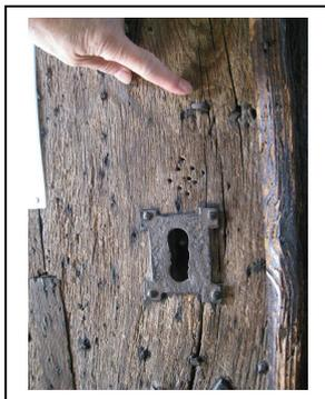
**Lock (probably 14C) nailed through the oak door and ends of nails clenched over — not removable without damage.**
