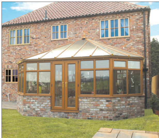
Figure 1 Victorian style conservatory roof
