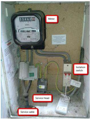
This is the most potentially dangerous part of your system. Fault currents could potentially reach into the 1000's of Amps, more than enough to start a fire or kill someone. As such it's not really something you should be poking around at, but here are some simple visual checks you can make.
