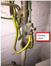
Bonding clamps are used on copper water and gas pipes. They aren't appropriate for the lead sheathing of the service cable. The locking screw can be forced through the sheathing and penetrate the cable creating potential fault currents into the 1000's of amps. Here is a picture showing the damage a bonding clamp can do. The centre of the rectangle is the paper wrap before you get to the live a neutral conductors. A lucky escape for this
