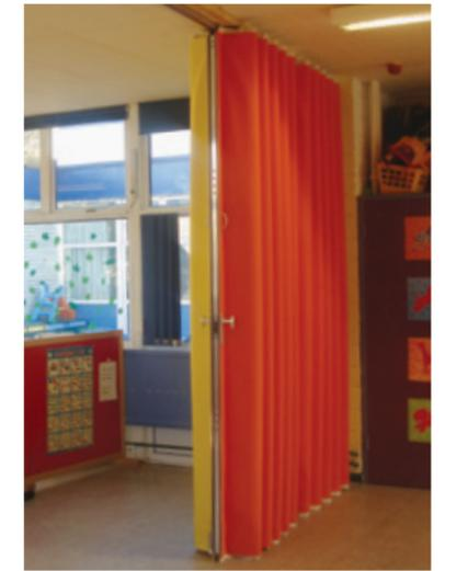
Folding partitions can run on tracks fitted flush to the floor or fitted directly to an existing floor finish.
